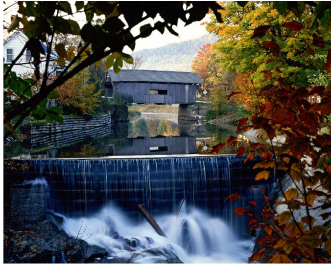
Covered bridge in Warren, VT. (Photo credit: Dennis Curran, Image Relay).
