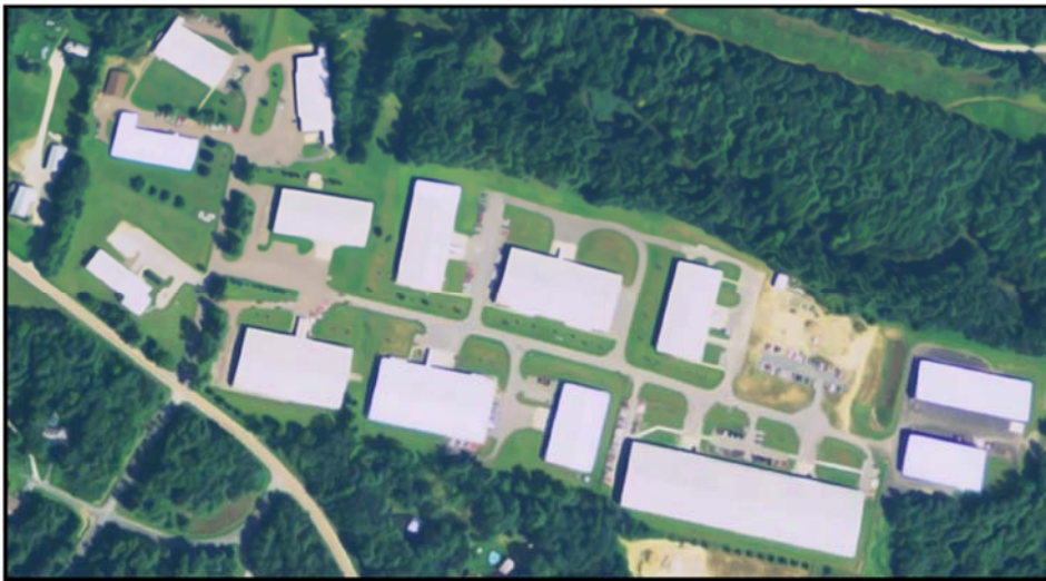
FIGURE 8: Efficient Use – Industrial Example
