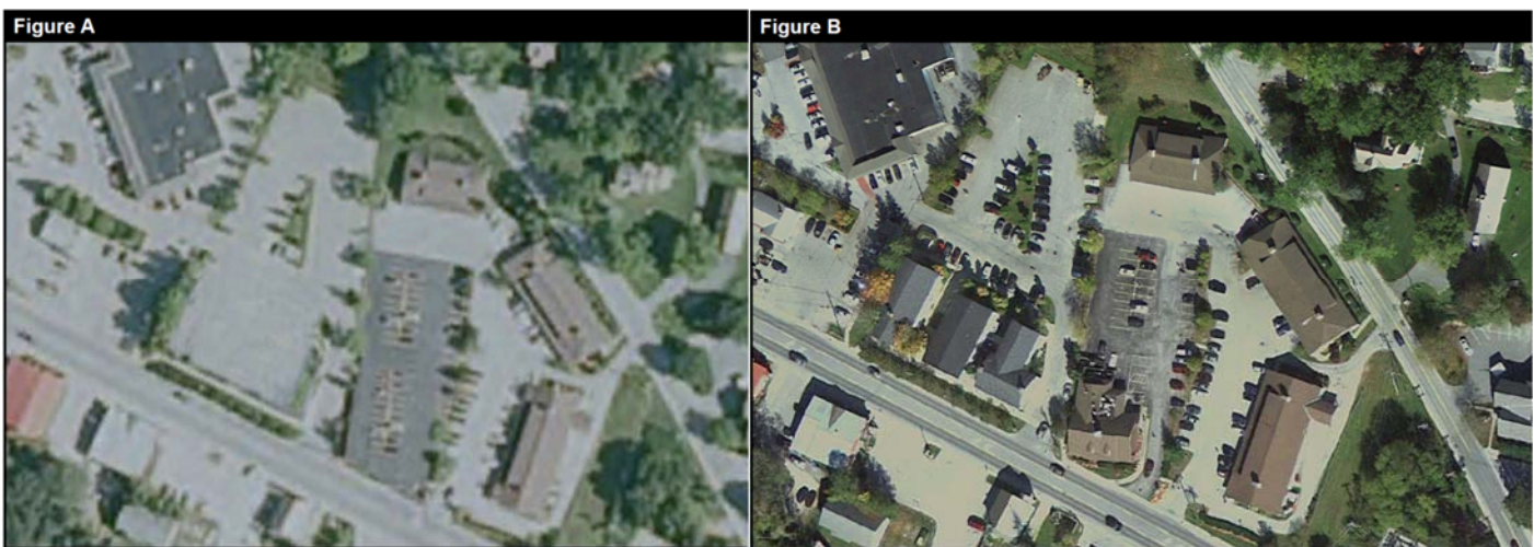
FIGURE 12 A & B: Infill project minimizing broad road frontage. Adding new multistory buildings to a large parking area in front of a strip mall breaks up broad road frontage and adds depth to the development.
